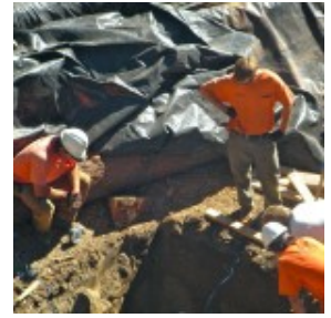
Working on the park's stormwater drainage system.Â Â Photo/Kathryn Reed
