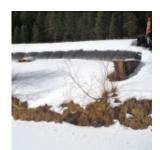
A water filled berm keeps the Upper Truckee River out of the new channel near Lake Tahoe Airport. Photo/Kathryn Reed
