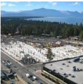
South Lake Tahoe convention center project in 2007. Photo/Provided
