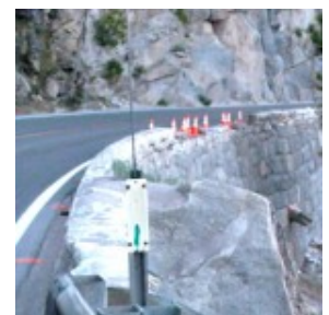
The rock wall at Echo Summit that will be replaced. Photos/LTN
