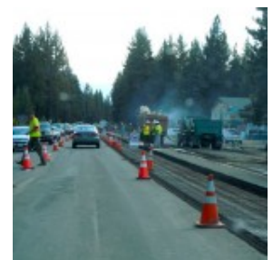
Construction season in South Lake Tahoe. Photo/LTN
