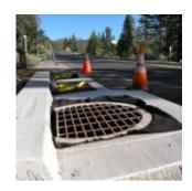
The project on Luther Pass will direct roadway water runoff to treatment collection facilities. The project also widened highway shoulders, constructed curbs and gutters, and repaired and constructed drainage facilities between the Alpine County line and Highway 50 in Meyers.
