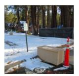
Looking toward the lodge from the lake, the round item at the bottom of the photo is where a hole was drilled, the concrete behind and to the left of the sign is an underground tank, and the fenced off area to the right is the sparge unit.
