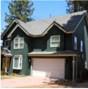
A house on one end of Fern Road.
