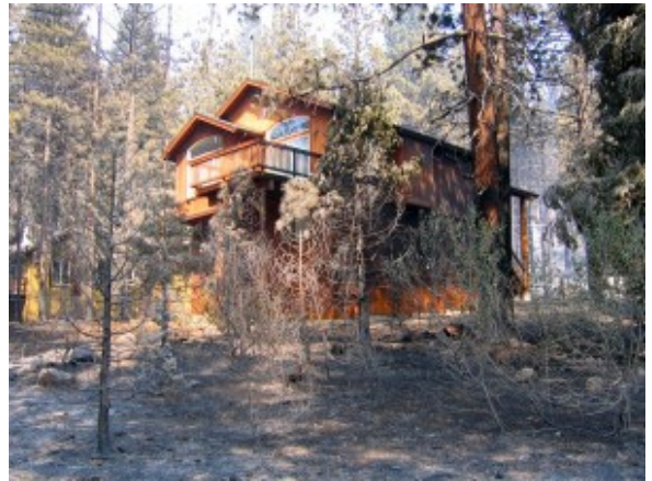
Proper defensible space spared this house in the Angora area. Photo/Lake Valley Fire
