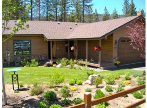
Houses in the Angora burn area were featured on a 2010 home tour. Photos/LTN
