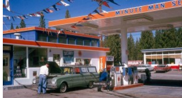
Highway 50 and Lodi Avenue in 1965.
