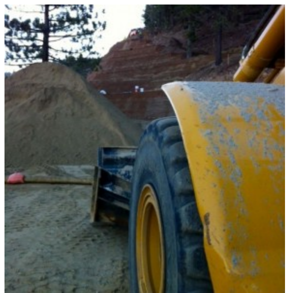
Heavy equipment and piles
