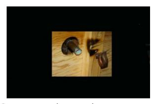
Damage done by copper thieves to a USFS bathroom on the South Shore. Photo/USFS
