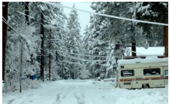
Power and cable lines are sagging in South Lake Tahoe.
