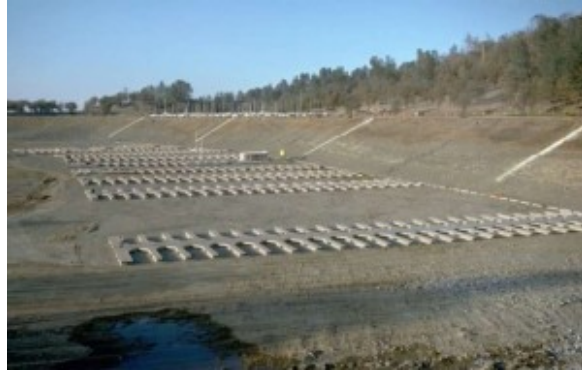
Boat slips in Folsom Lake during the 1976 drought. Photo/California Department of Water Resources
