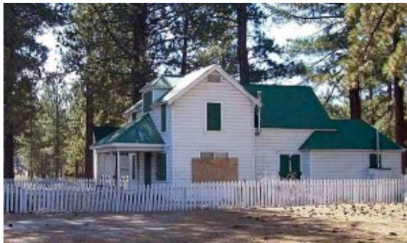
Boarded up Barton Ranch building in South Lake Tahoe. Photo/Bill Kingman
