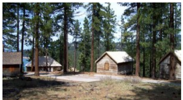
Round Hill Pines is being renovated. Photo/Bill Kingman
