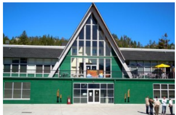
Lake Tahoe Airport doubles as city hall.
