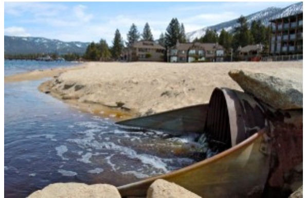
Water from the Bijou area drains from a large pipe right into Lake Tahoe. Photo/LTN file
