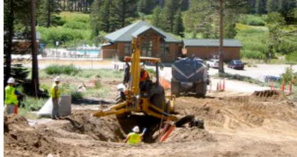
Kirkwood power house being built after the 2010 fire. Photo/Provided
