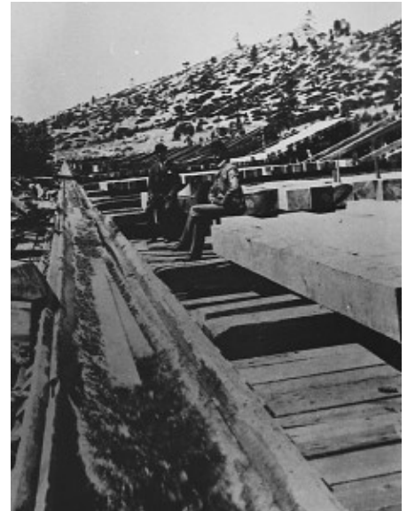
Flumes eased the transport of logs.
