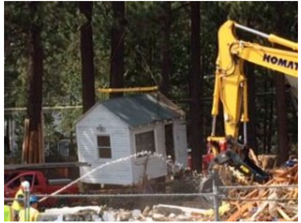
The old cabin is being relocated. Photo/Dave Kurtzman
