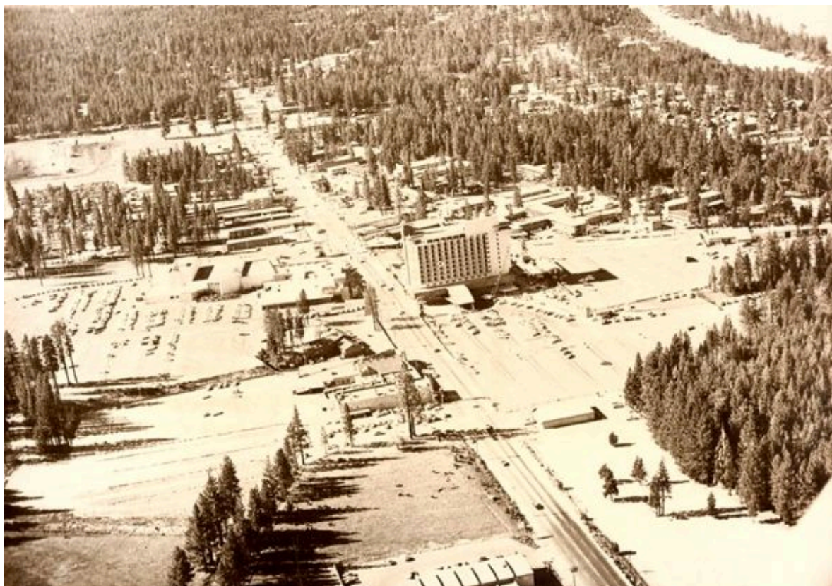
An aerial view of Stateline in 1962. Photo/UNR Special Collections Department
