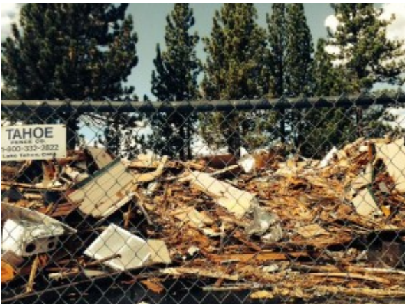
The pile of debris.
