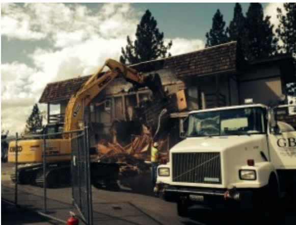
The building being razed Sept. 15. Photo/Provided
