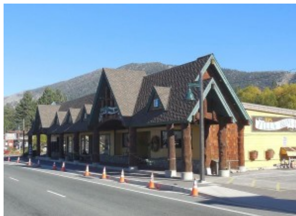
This South Tahoe building was remodeled about 10 years ago. Photo/Bill Kingman
