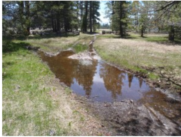
Before the work began the trail was impassable. Photo/California State Parks
