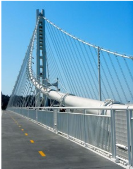
The foot path adjacent to the new section of the Bay Bridge.
