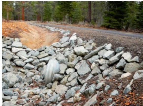
Erosion control measures line the trail.
