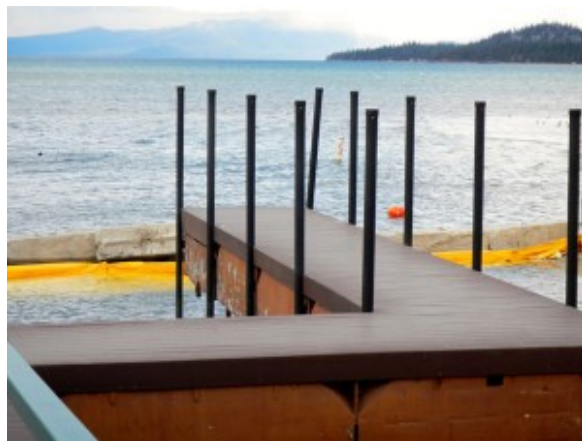
Prep work at Ski Run Marina in anticipation of dredging. Photo/LTN
