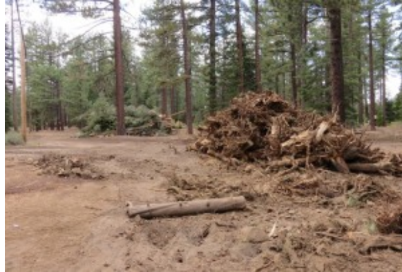
Tree removal this summer at Camp Richardson. Photo/Liana Zambresky
