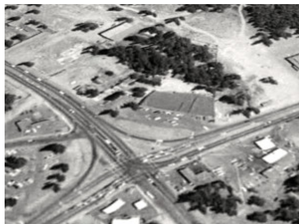
Not much development existed at the Y in 1969. Photo/U.S. Geological Survey
