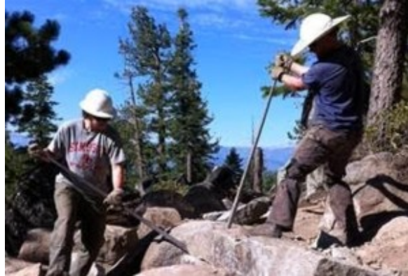
Crews work on a multi-use trail in Stateline. Photo/Provided
