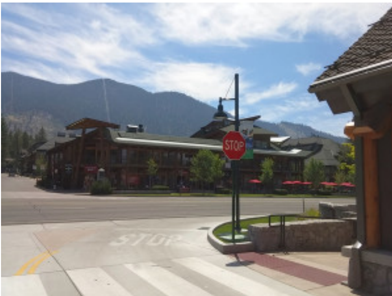
Poplar at Highway 50 is now a driveway to parking.
