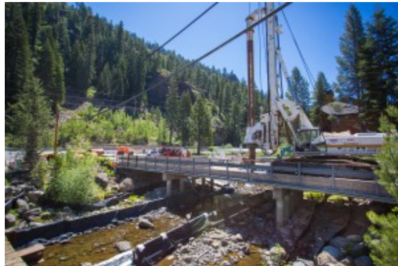
Alpine Meadows Bridge replacement. Photo/Erik Bergen
