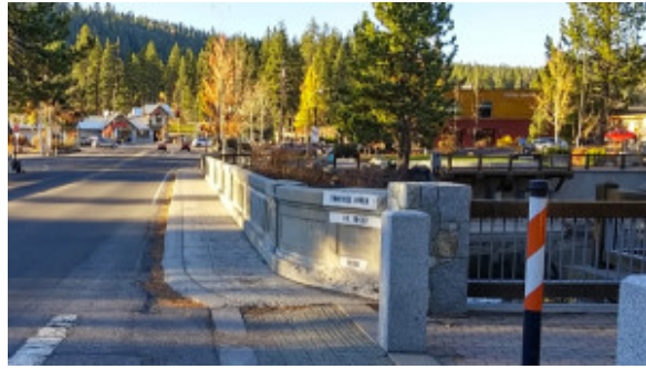
Fanny Bridge in 2015 with its expanded Y intersection and islands. Photo/Bill Kingman
