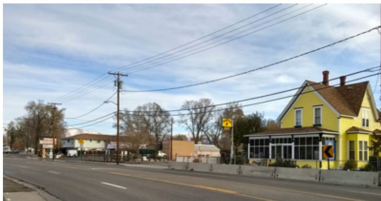
That same building still stands today. It is Frontier Antiques.
