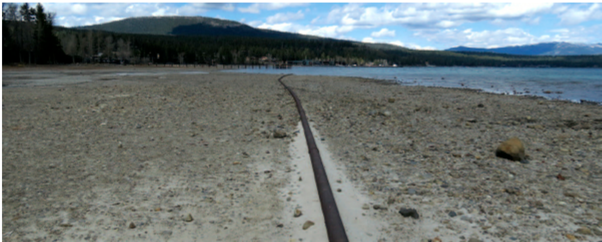
The beach with the exposed pipe.
