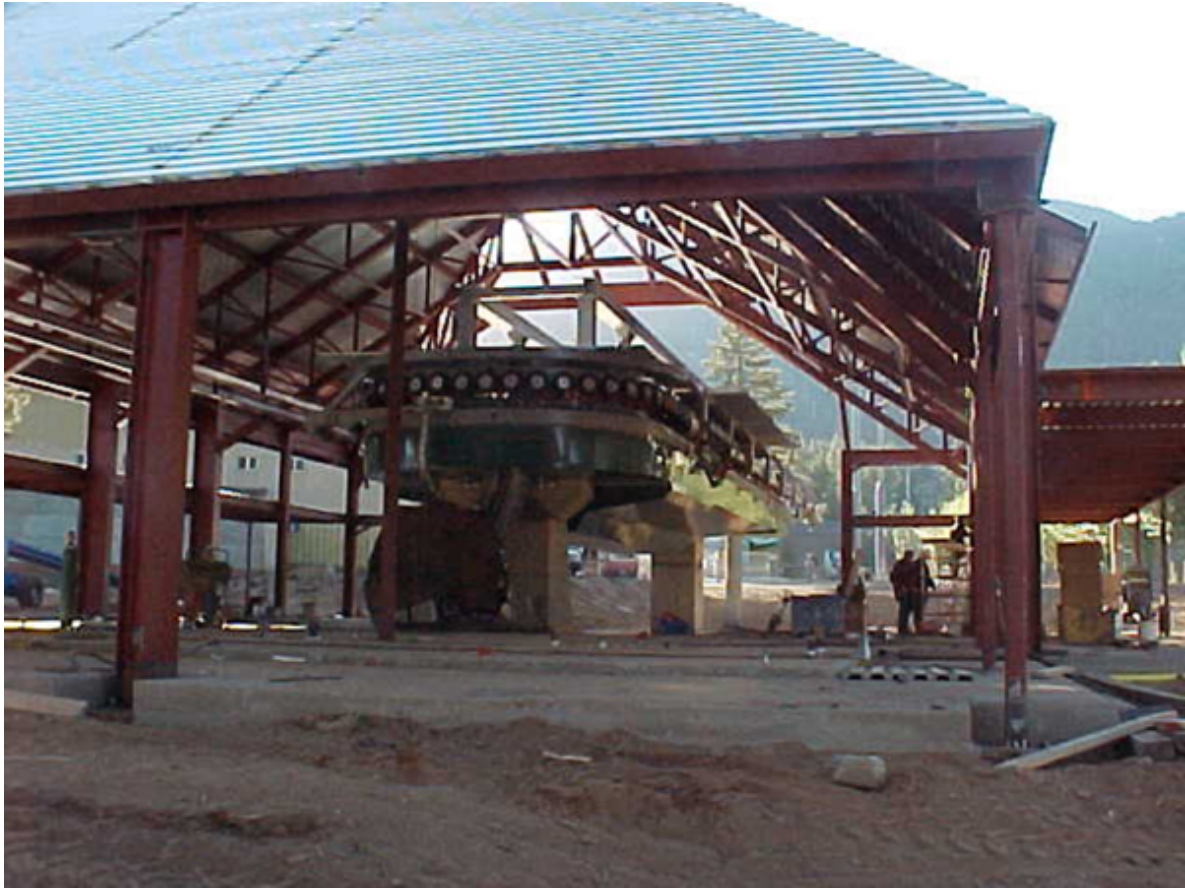
The gondola under construction. Photo/Heavenly Mountain Resort
