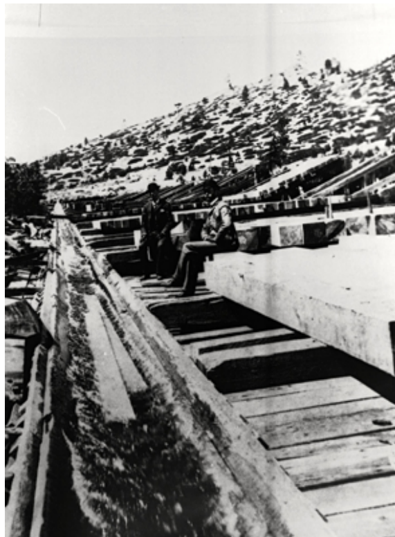
Flumes were used as one form of transport of logs harvested in Tahoe.
