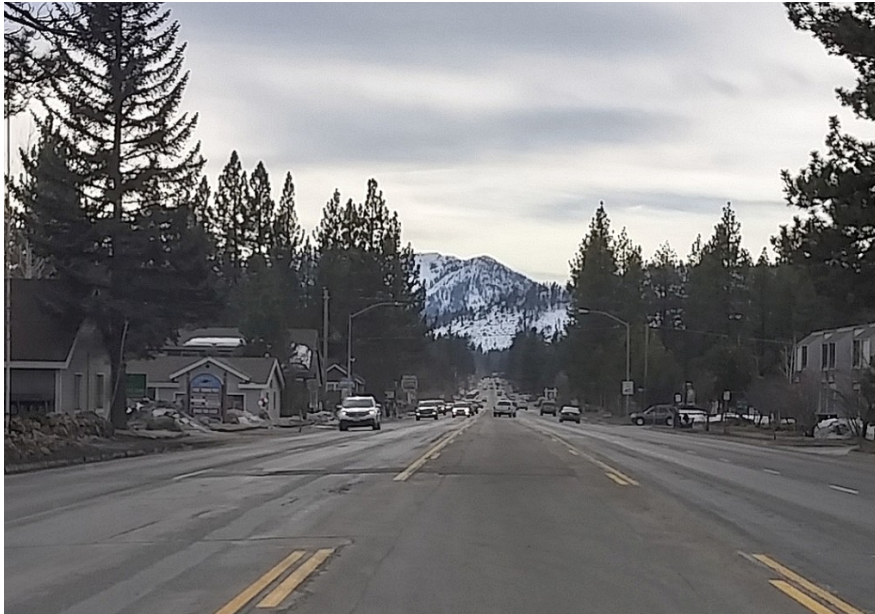
Highway 50 at Stockton Avenue in South Lake Tahoe in 2016. Photo/Bill Kingman
