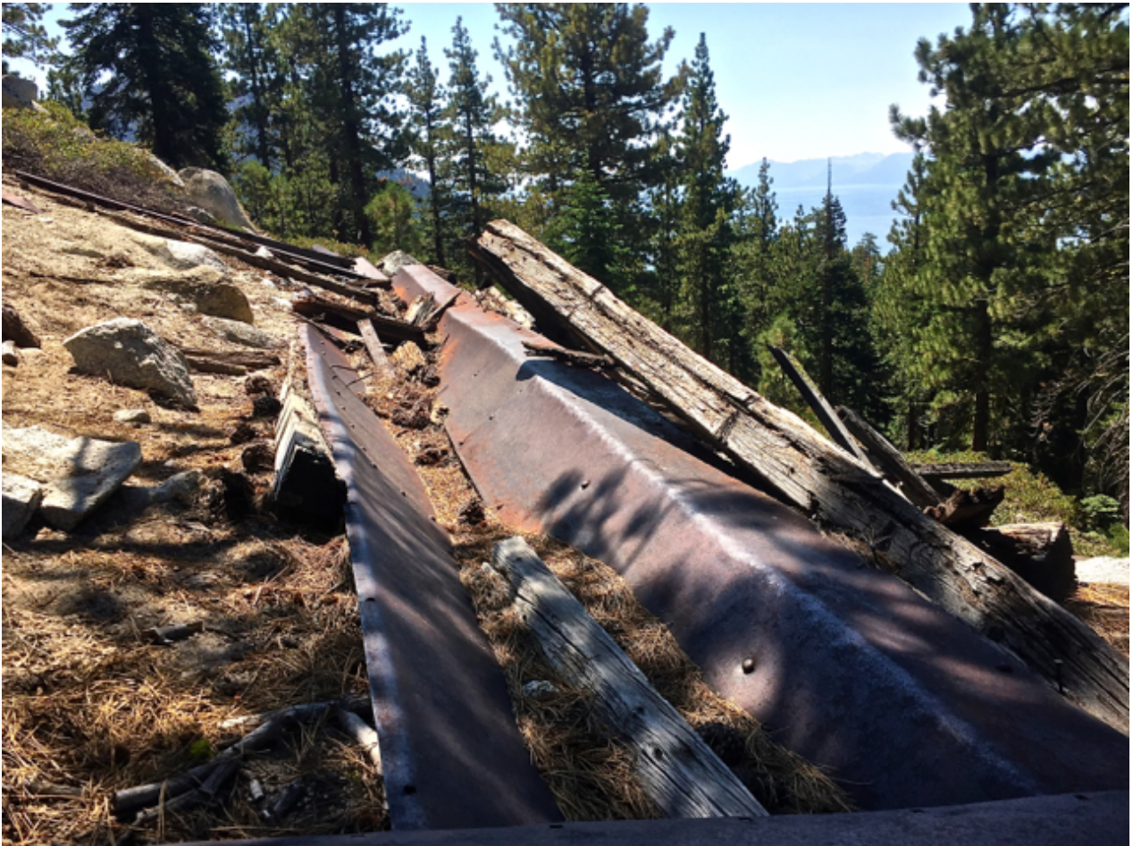
The V flume took logs through the mountains for the mines in Virginia City. Photo/Kathryn Reed
