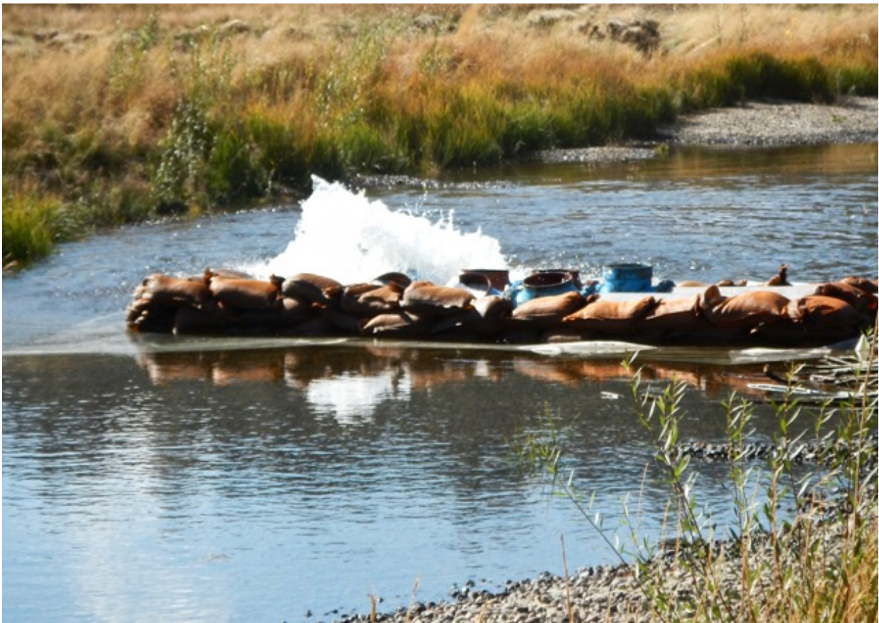
Water is being pumped into the new channel. Photo/Kathryn Reed
