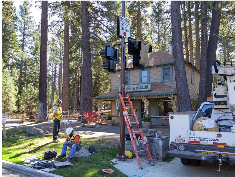
A pedestrian light is being installed at Camp Richardson. Photo/Bill Kingman
