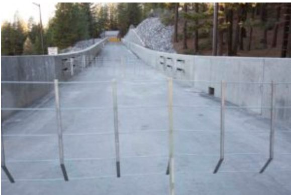
Mount Rose truck ramp today. Photo/Provided
