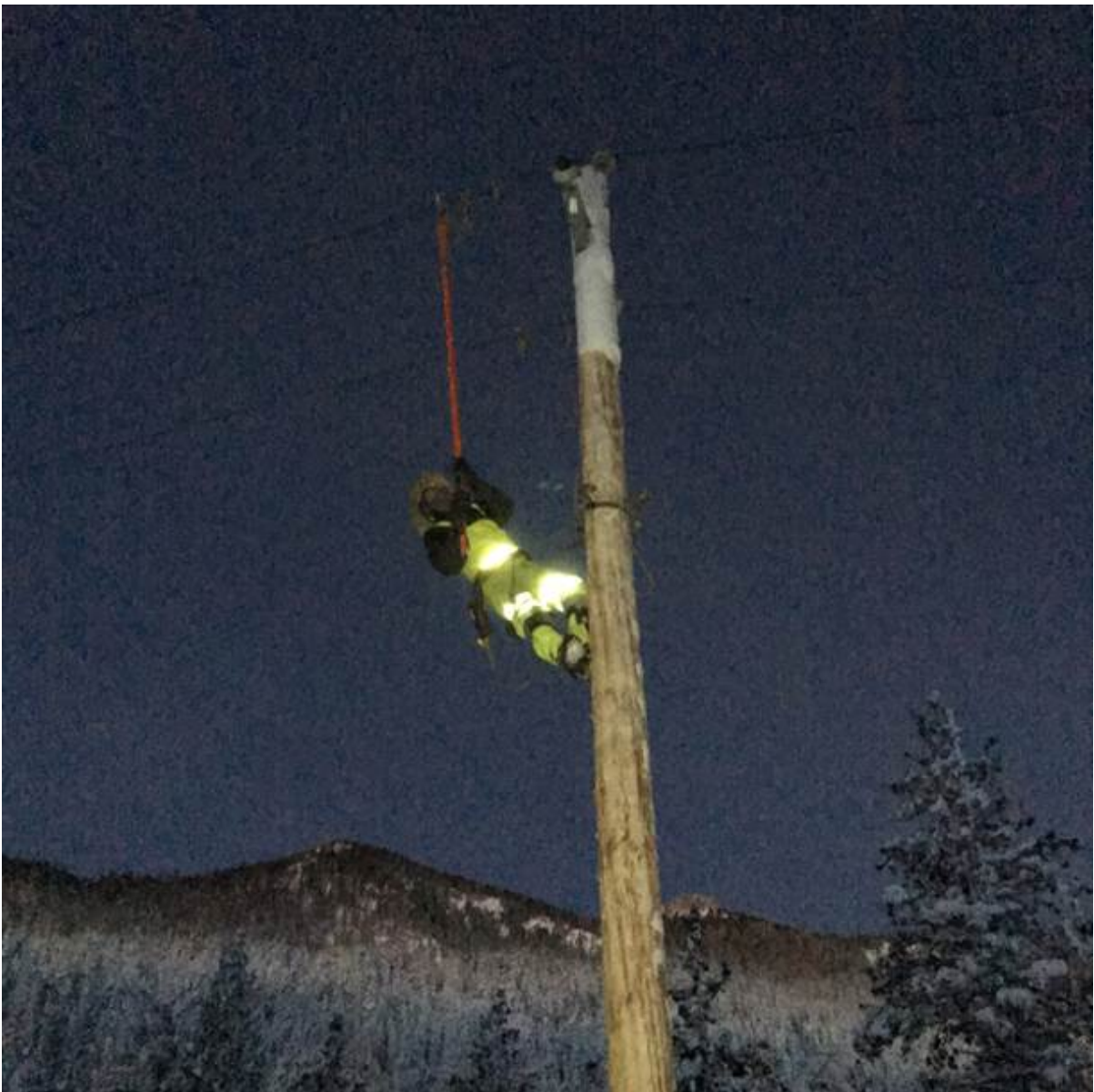
Liberty Utilities crews work at all hours to restore power. Photo/Provided
