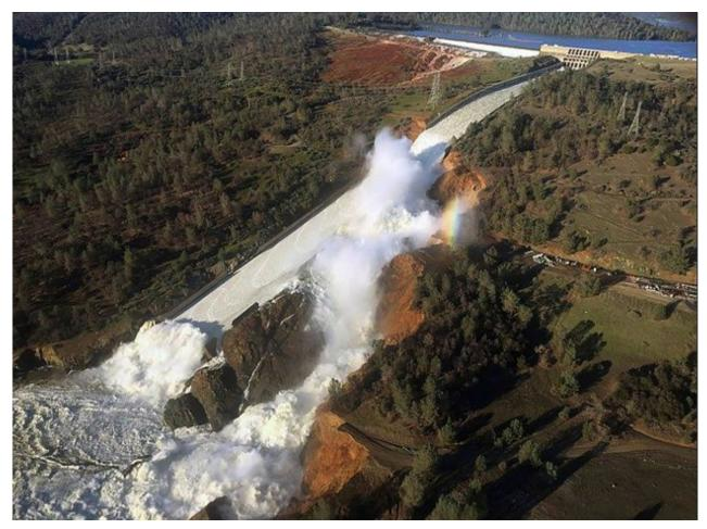
Water flowing from the eroded overflow spillway of Oroville Dam in February. Photo/California Department of Water Resources
