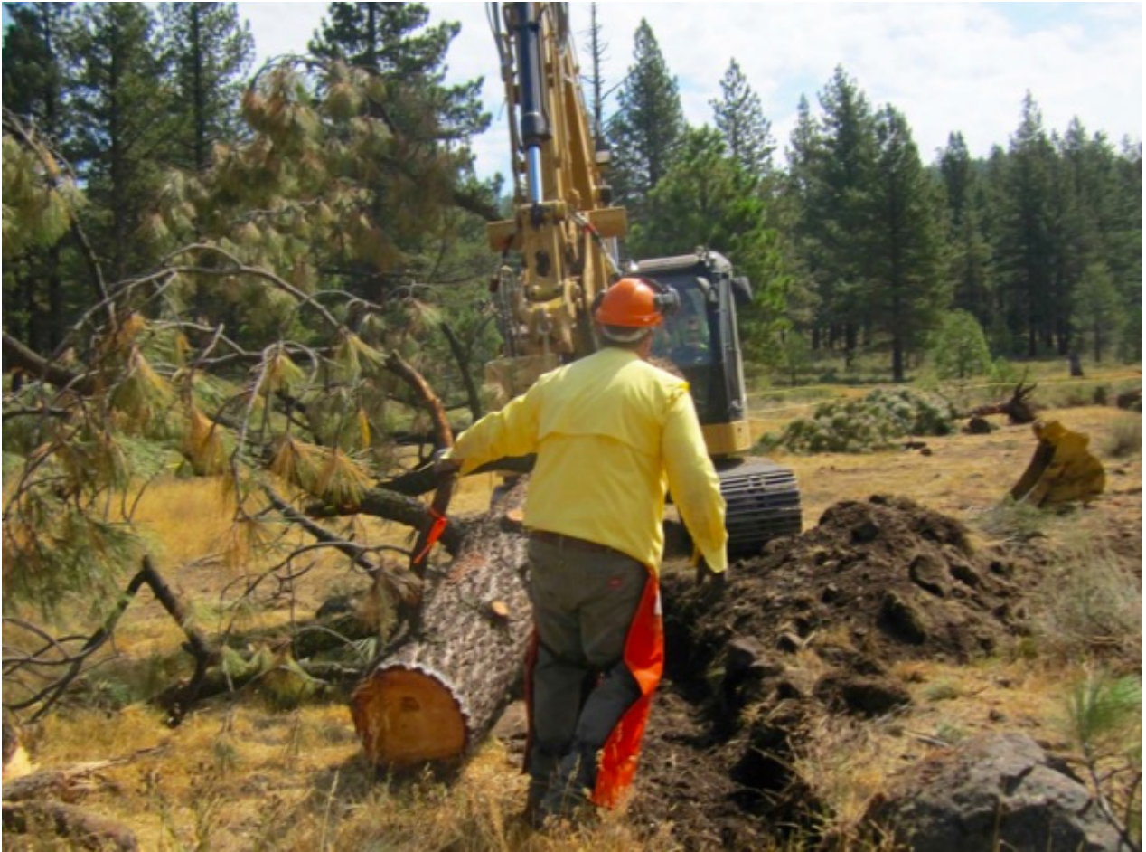
Crews work to restore meadows throughout the Sierra Nevada. Photo/Beth Christman
