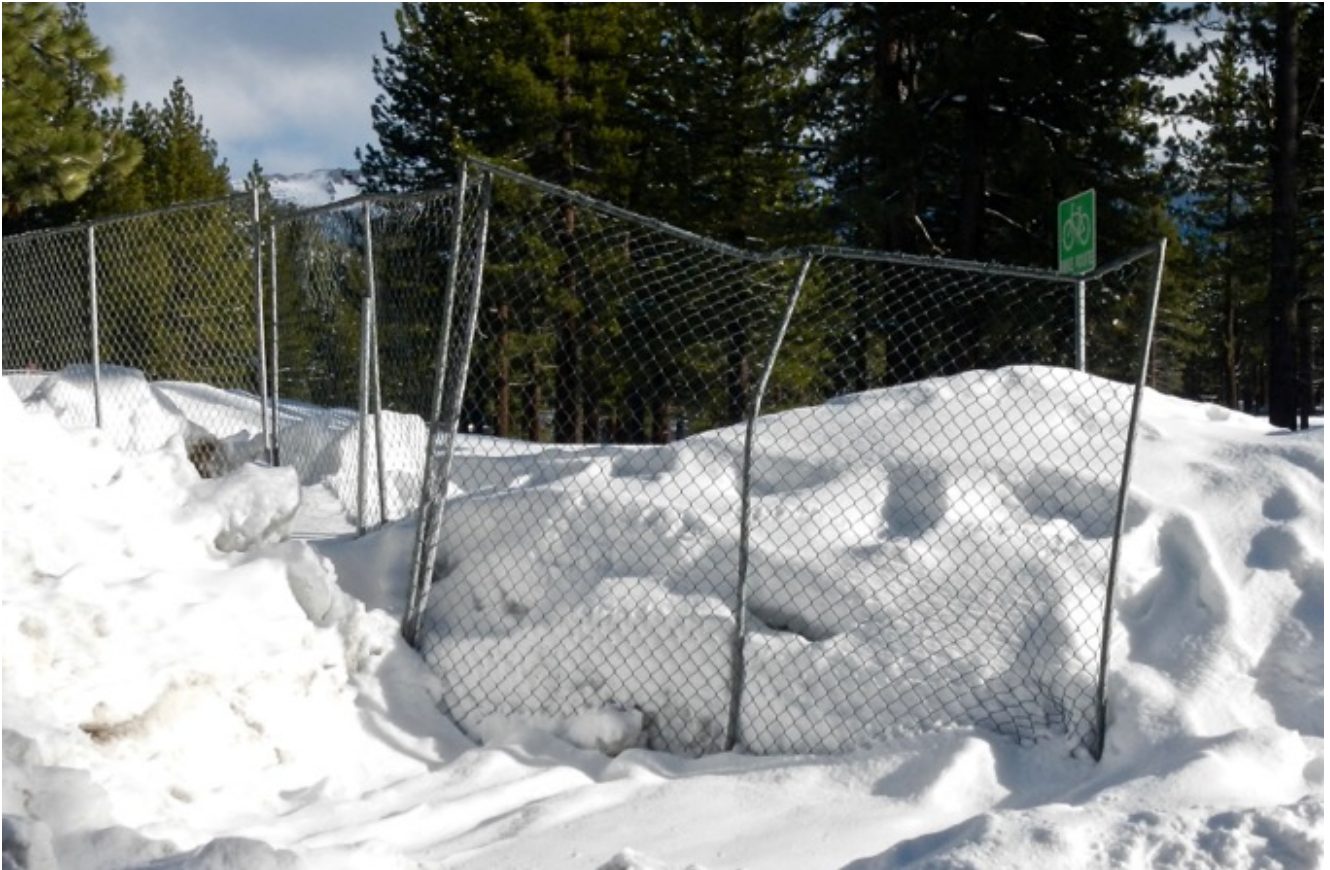
Damaged chain link fences remained for months after SnowGlobe. Photo/LTN
