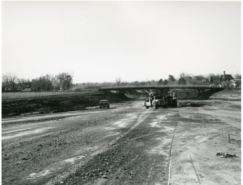
Building Interstate 80 near Reno in May 1972. Photo/NDOT
