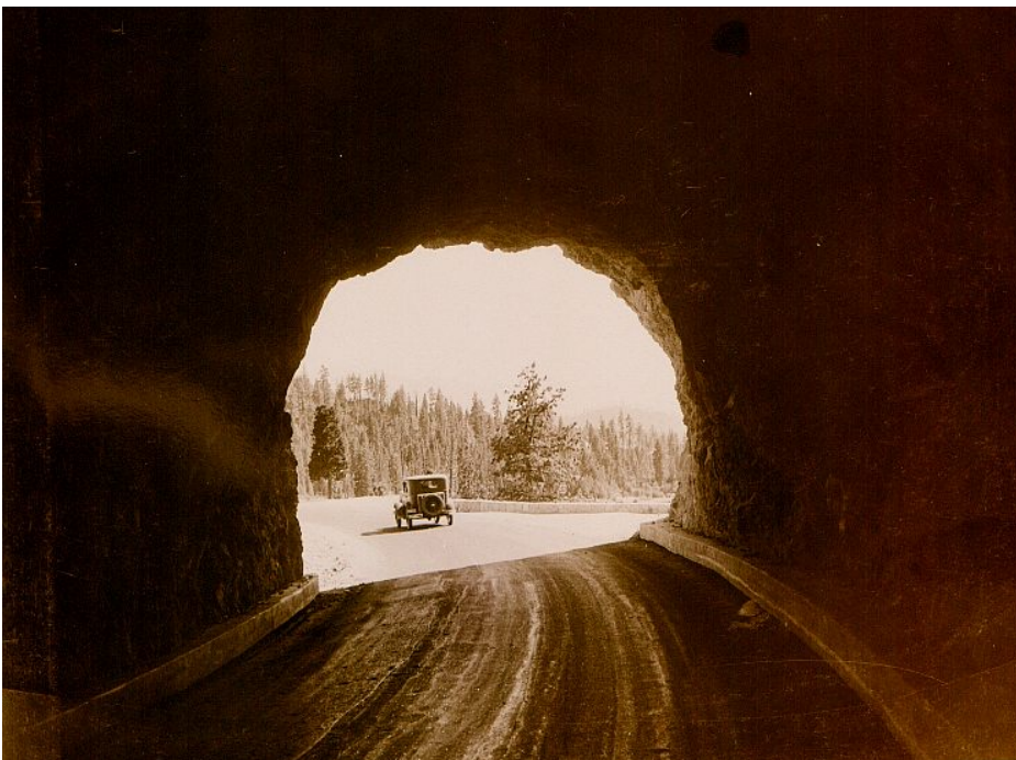
Cave Rock tunnel, circa 1930s. Photo/NDOT
