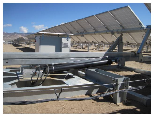
Hydraulic pistons adjust banks of panels about every five minutes. Photo/Bonnie Turnbull
